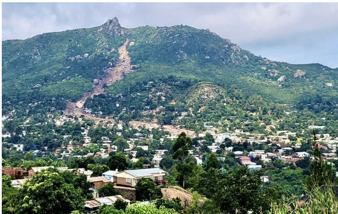
Photo 6.2: Debris Flow in Soche Mountain, Blantyre City, Malawi, during Tropical Cyclone Freddy, 2023
