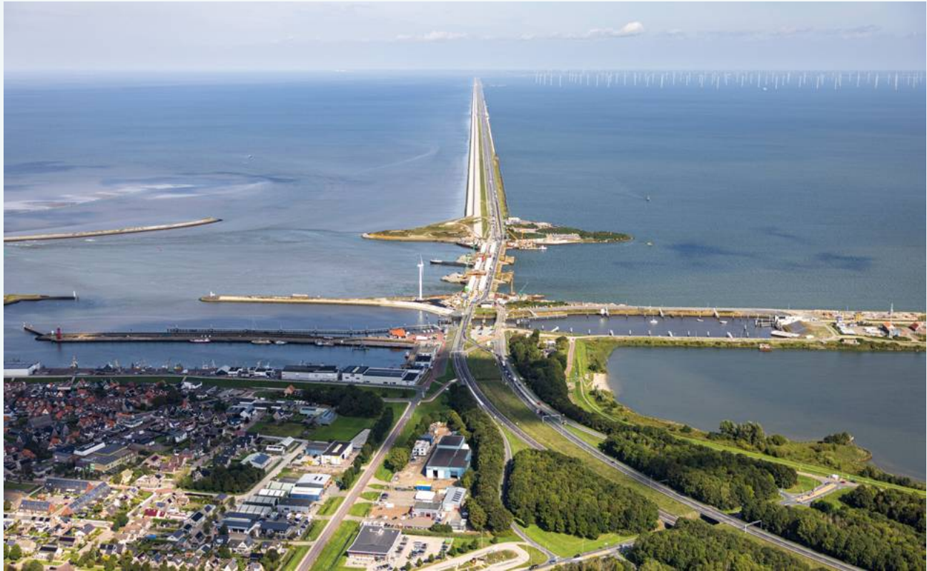
Photo B2.2.2: Flood Defense Structure. Longitudinal view on Afsluitdijk, North Holland
