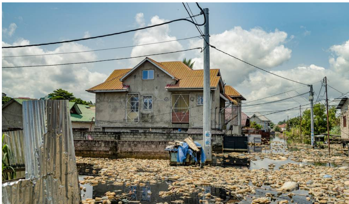
Photo 5.3: The Aftermath of Floods in Kinshasa, Democratic Republic of Congo, 2024
