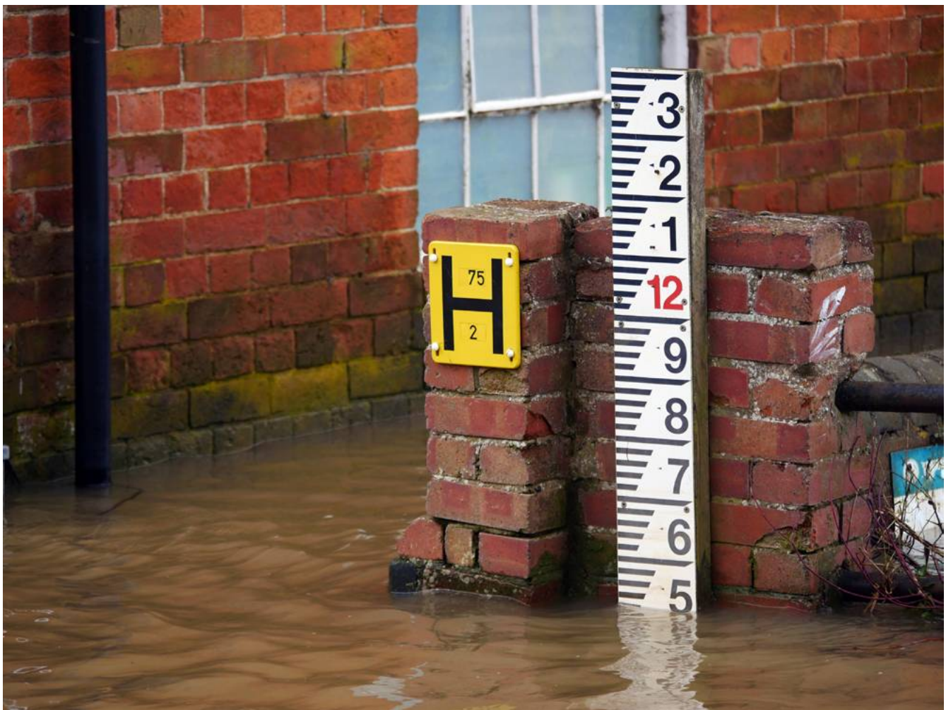
Photo 5.1: Water Level at the Flooded Abbey Mill in Tewkesbury, England
