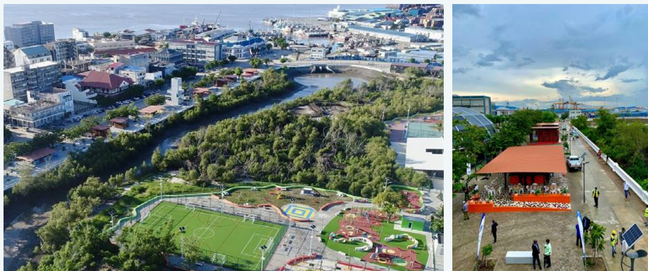
Photo B1.1.1: Chiveve River Green Infrastructure Project
