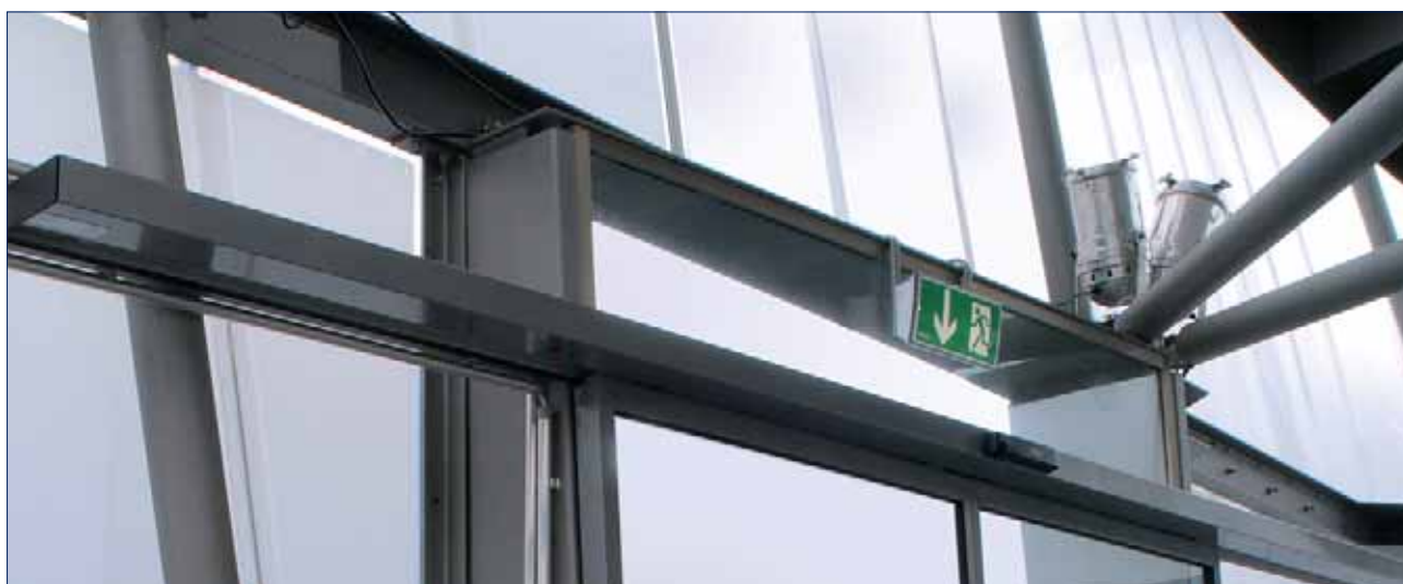
BBI Tower Airport Berlin, Germany
