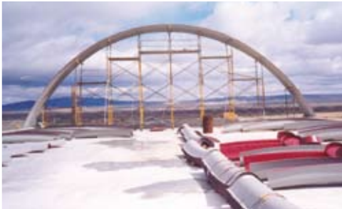
Andamios Scaffoldings Echafaudages
